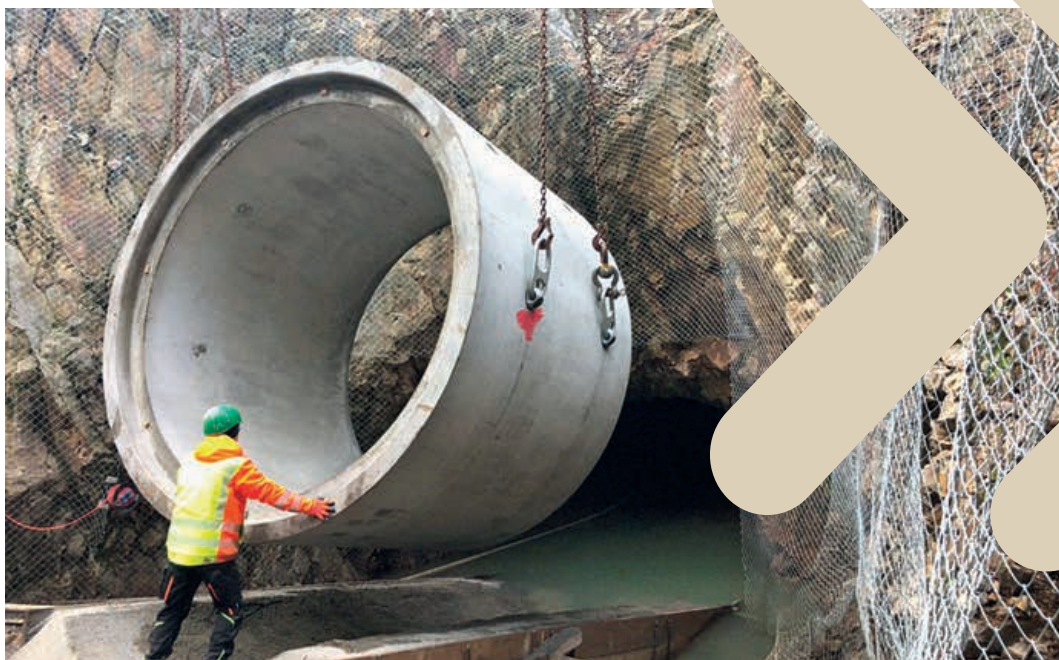
A logistical tour de force: the installation of the multi-tonne shaft rings
